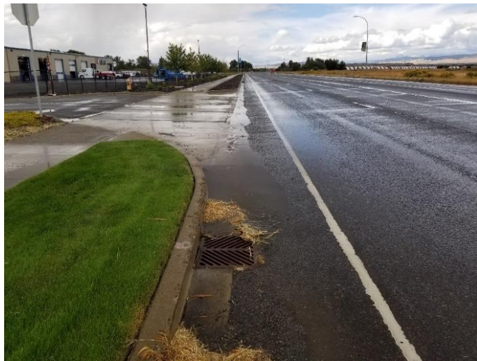
Figure 3.9 Approaches contribute runoff to catch basins
