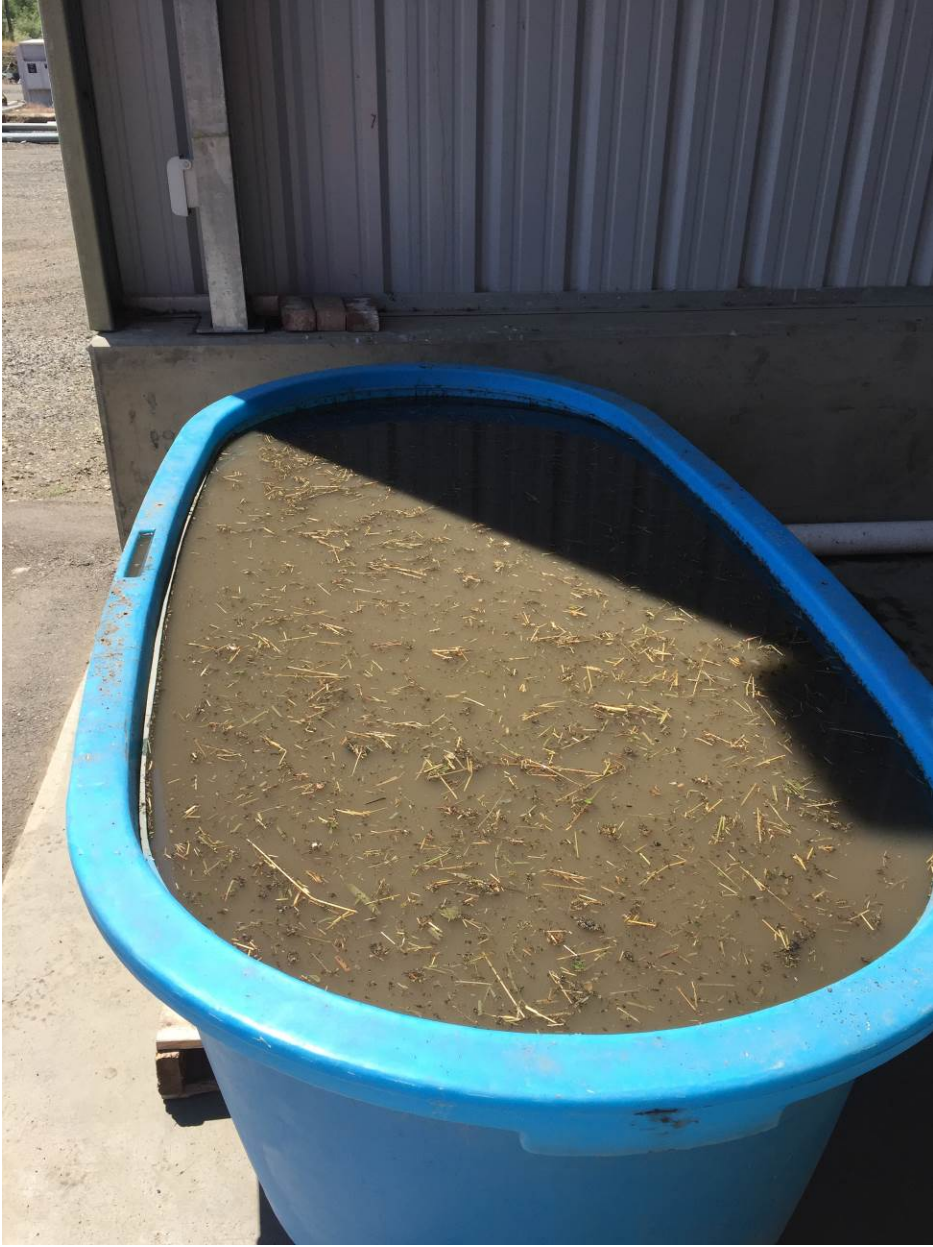
Material collected during catch basin cleaning. Appeared to fill the basin to almost the same depth as in April. Smelled horrible. No dead mice observed.
