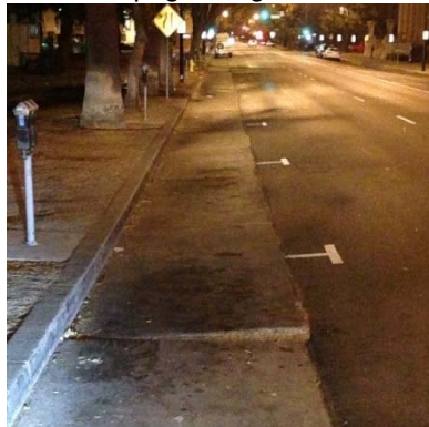
↑ A lifted concrete slab along the Central Business District route during scheduled street sweeping on August 20, 2015.
