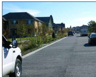
Porous Concrete – low volume residential street
